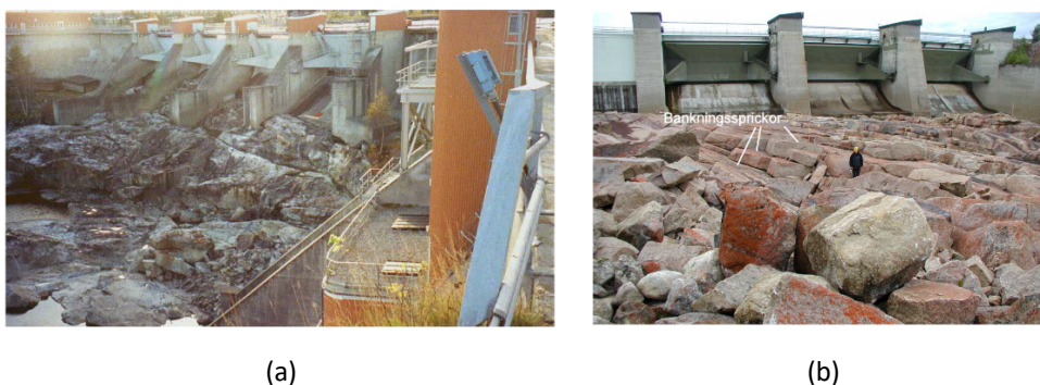
Figure 1-1: Erosion of rock channels (a) Midskog dam (Billstein et al., 2006), (b) Harsprånget dam (Mörén, 2005).
